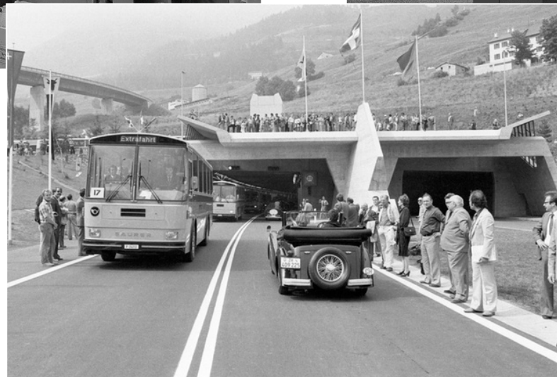
Gotthard Road Tunnel 1980
